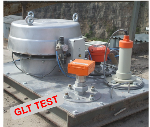
A Typical Silo Protection installation with Ground Level Test, plus an additional contents gauge
